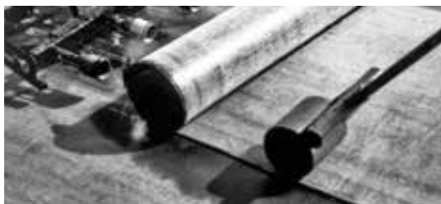
Figure 9: Heat welding installation of Derbigum
