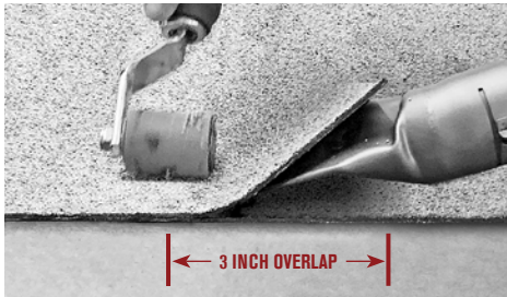
FIGURE 7: Stitching the overlap
