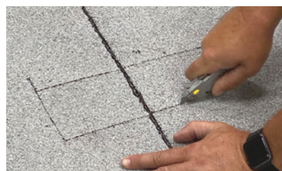
FIGURE 2: Minimum 2" wide test cuts should be slit across the welded seam
